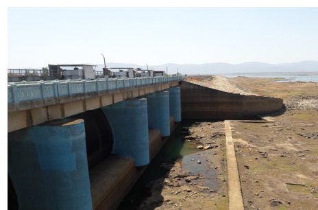
Gohira Irrigation Project (Photograph taken during Rabi Season)
